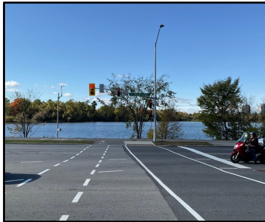
Figure 8. Street lighting is provided for arterial roads but walking paths have limited to no lighting.
